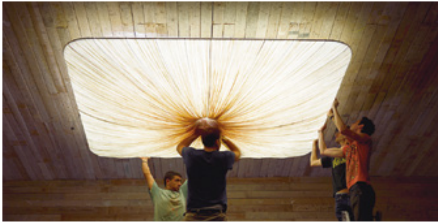
Test installation of Custom Nara 240cm / 94"
