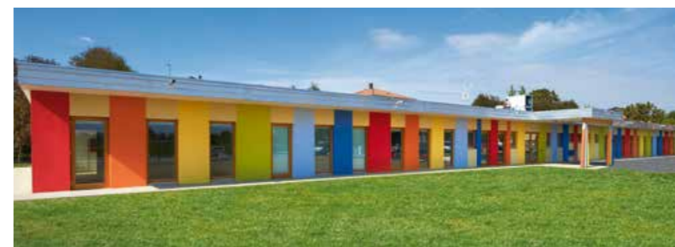
School „Garibaldi“ in Soliera, Modena (I)
