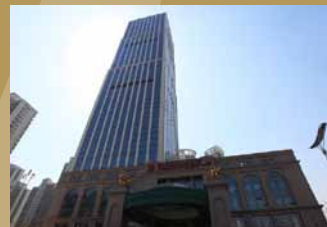
Zhongnan International Plaza Hotel in Nantong, China
